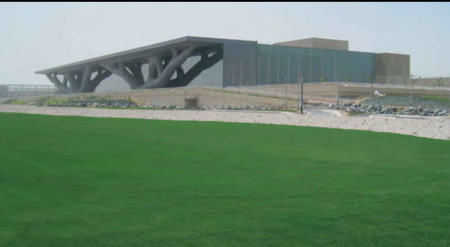
Qatar Convention Centre Doha (Qatar)
